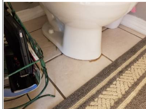
Toilet bowl loose in master bathroom during time of inspection - recommend securing to floor and caulking around the base
